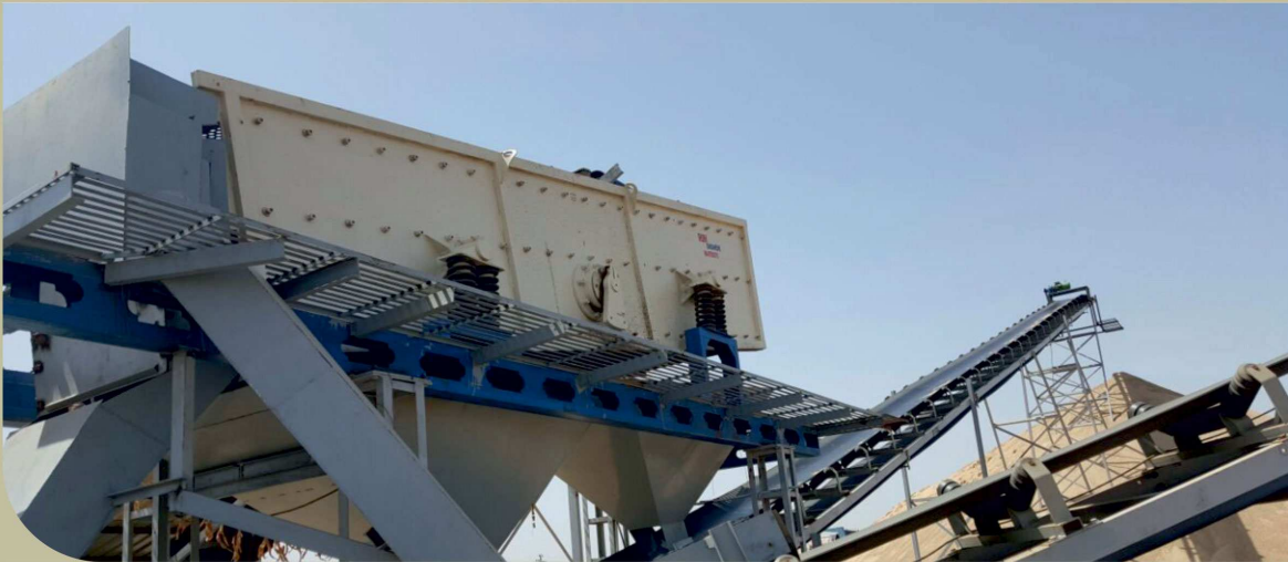
Sand screening plant with conveyor system
